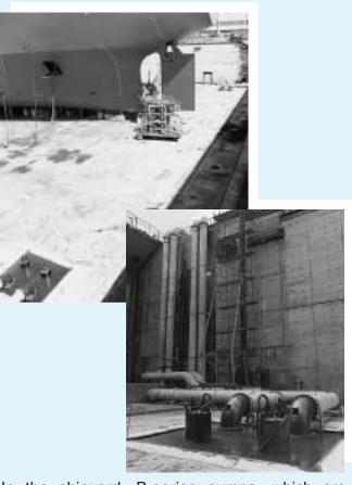
In the shipyard, B-series pumps, which are operated by fully-automatic control, work for level control and dry up. For sea water, sacrificial anodes are applied.
