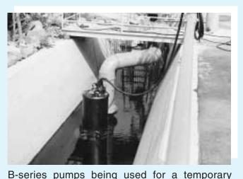
installation during rainy season. It is used to pump up water of branch river to the main stream when the water level of main stream becomes higher than that of the branch river.
