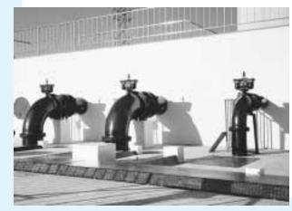
As it is silent during operation owing to its underwater operation, B-series pumps are often used at the basement of buildings in the city area.
