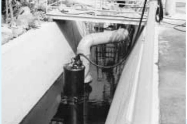
B-series pumps being used for a temporary installation during rainy season. It is used to pump up water of branch river to the main stream when the water level of main stream becomes higher than that of the branch river.
