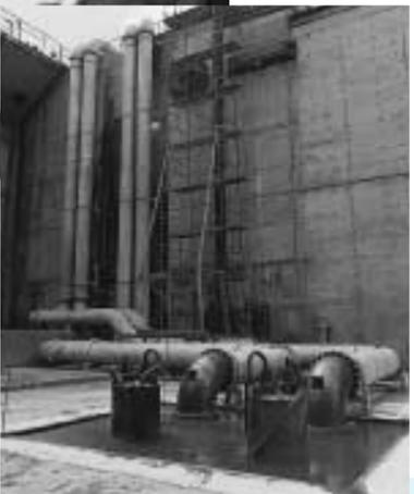
In the shipyard, B-series pumps, which are operated by fully-automatic control, work for level control and dry up. For sea water, sacrificial anodes are applied.
